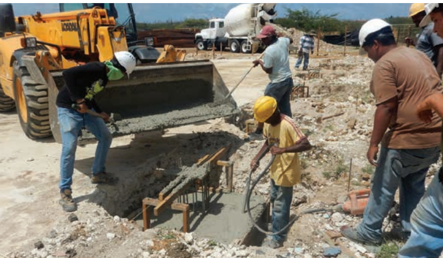
Two trainees (wearing white helmets), pouring concrete for the foundation.
